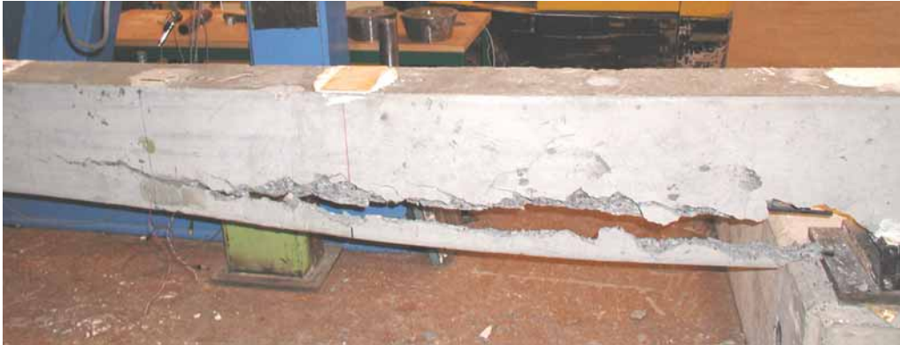
FIG. 15. Anchorage failure in the concrete for BMstat .
