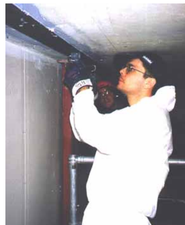
Figure 4-4: Bonding of laminate
