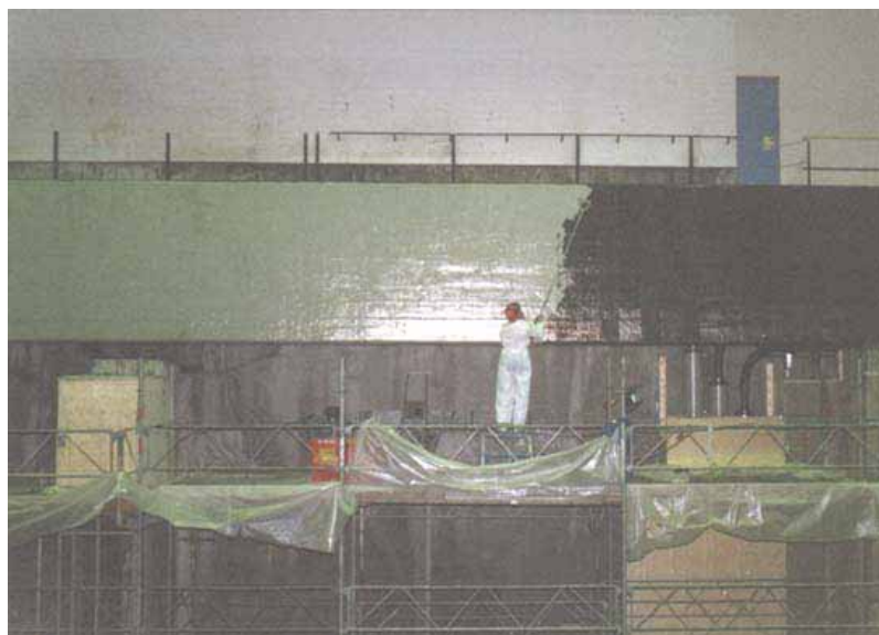
Figure 4-15: Finishing work on one of the beams
