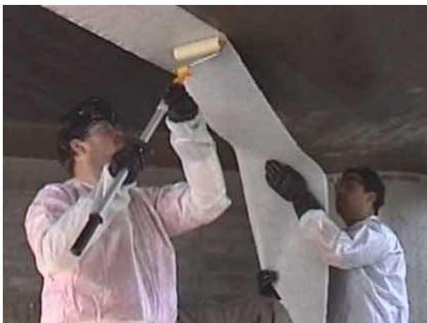
Figure 4-3: Hand lay-up. The light colour shows paper to be removed, Täljsten and Carolin (1999)
