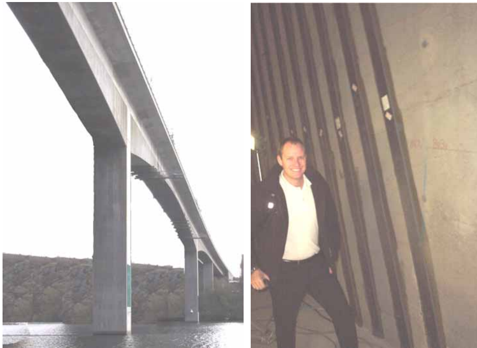
Figure 4-13: Gröndal Bridge. Outside (left), Inside (right).
